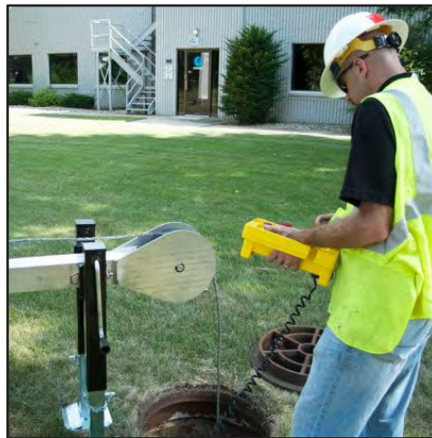
Figure 7. Use Joystick to Increase the Pullback Speed
