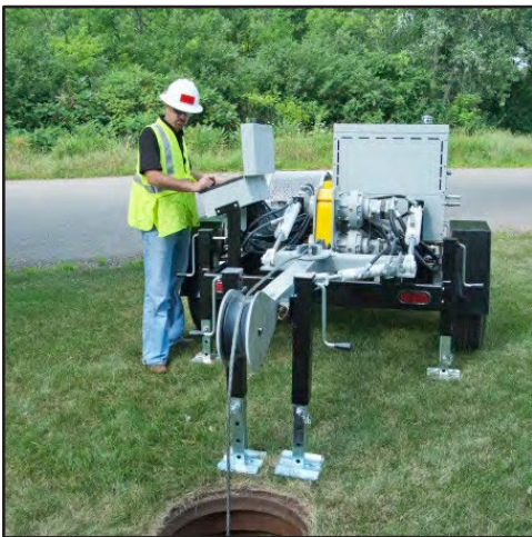
Figure 6. Monitor Pulling Tension and Distance
