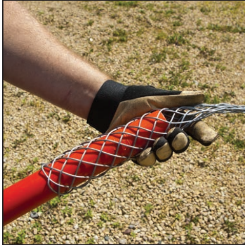
Figure 35. Install Pulling Grip on Conduit
