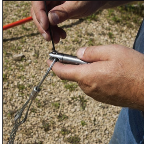
Figure 47. Install Swivel on Cable Grip
