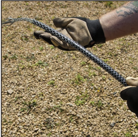
Figure 46. Install Cable Grip on Fiber Optic Cable
