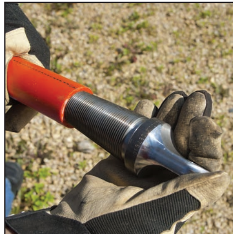
Figure 7. Installing Conduit Pulling Eye
