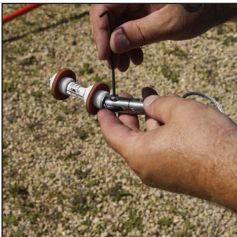
Figure 48. Install Carrier
