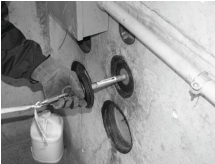
Figure 6 Attach Measuring Tape to Carrier and Insert into Duct
