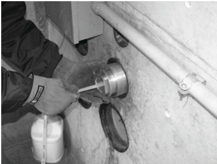
Fig. 8 Insert Threaded Adapter into Duct
