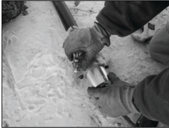
Figure 7 Close and Secure Winchline Blower Body
