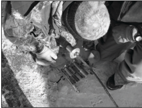
Figure 3 Place Threaded Adapter into Duct
