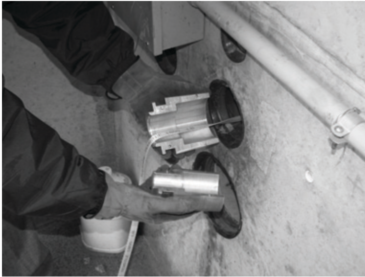
Fig. 7 Insert Threaded Adapter into Duct
