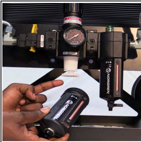
Figure 12. Check Fan Motor Moisture Separator Filter
